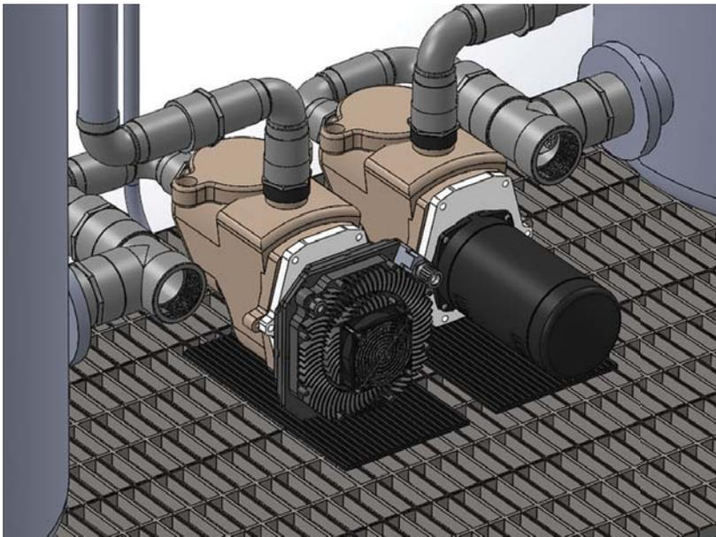
Comparing a conventionally installed motor (right) to a PCB Stator installation (left). *ECM PCB Stator Tech*
