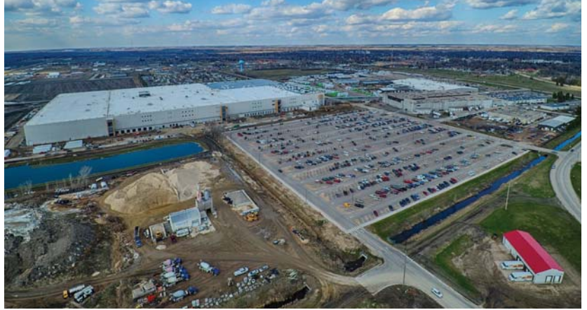
The PDCE building was designed by Minnesota-based Widseth, and McShane Construction served as general contractor on the project.
