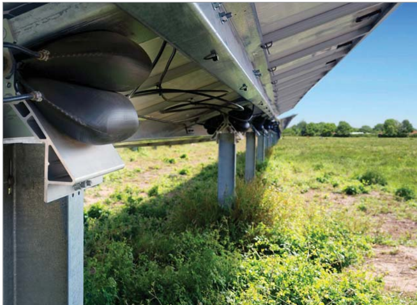
The Sunfolding T29 drive uses bladders to lift and aim solar panels.
