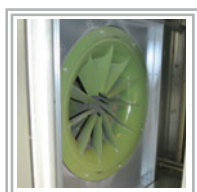
Pre- and Post-filtration: Intake and Exhaust. Two direct drive centrifugal fans with 2 sets of 10 bag filtration for each.
