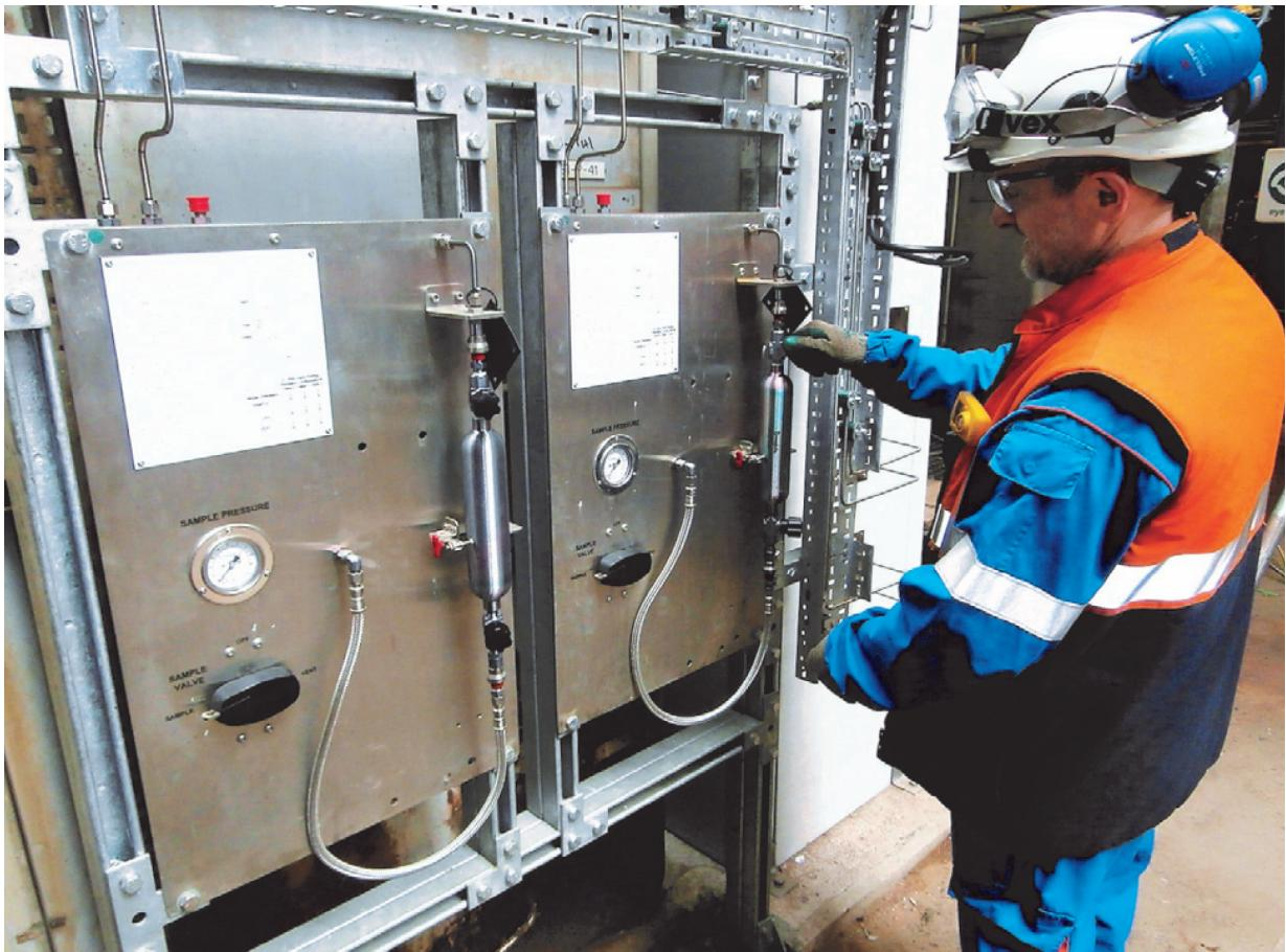
**Figure 1. With grab sampling, operators extract a sample from a fluid system and take it away for remote laboratory analysis. Images © 2022 Swagelok Company**
